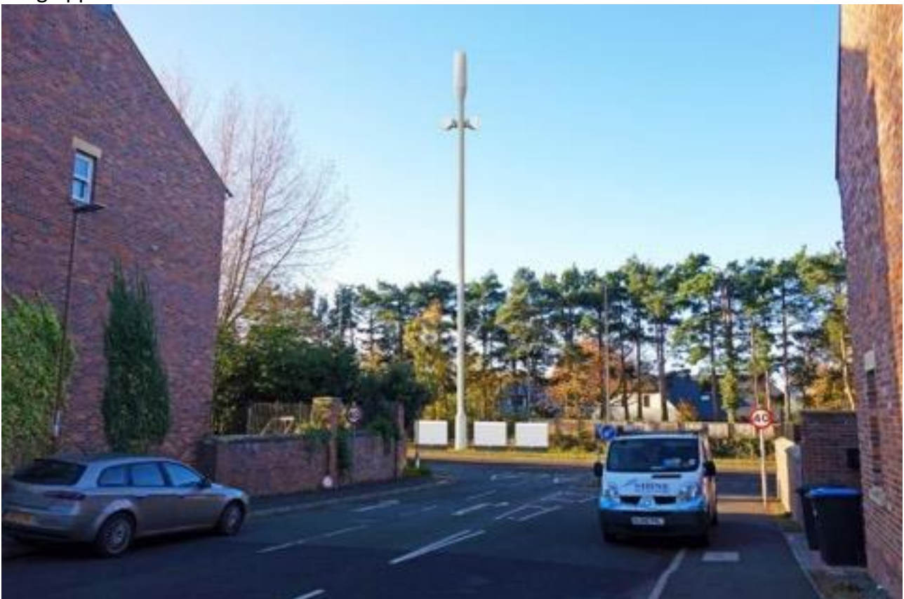
Example of a 20 metre phone mast.
